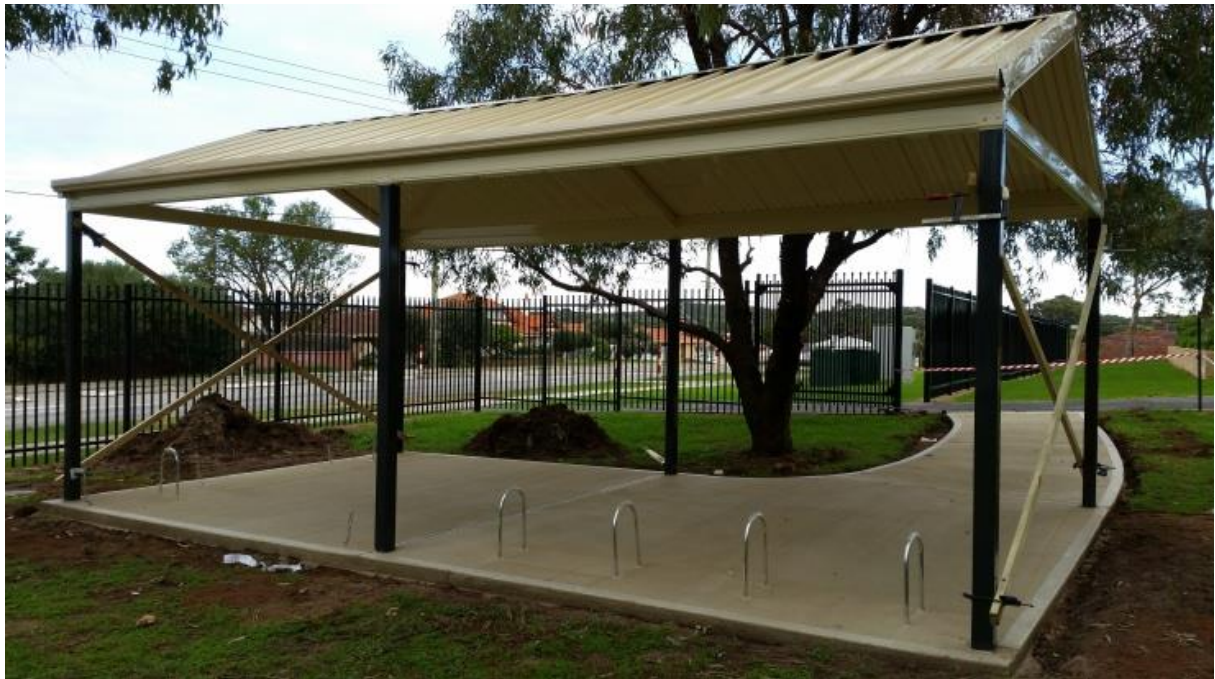
Phoenix Primary School's covered bike parking facility
